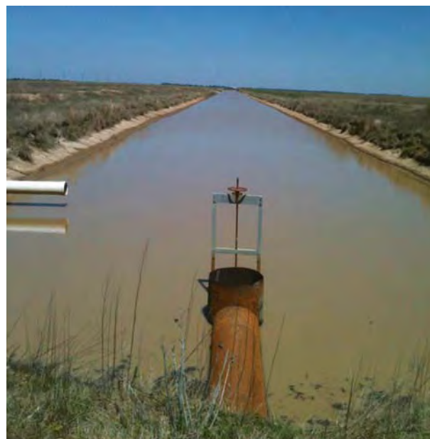
Photo 10-5. A typical tailwater recovery ditch.
