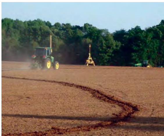
Photo 10-2. Surveying levees in a rice field.
